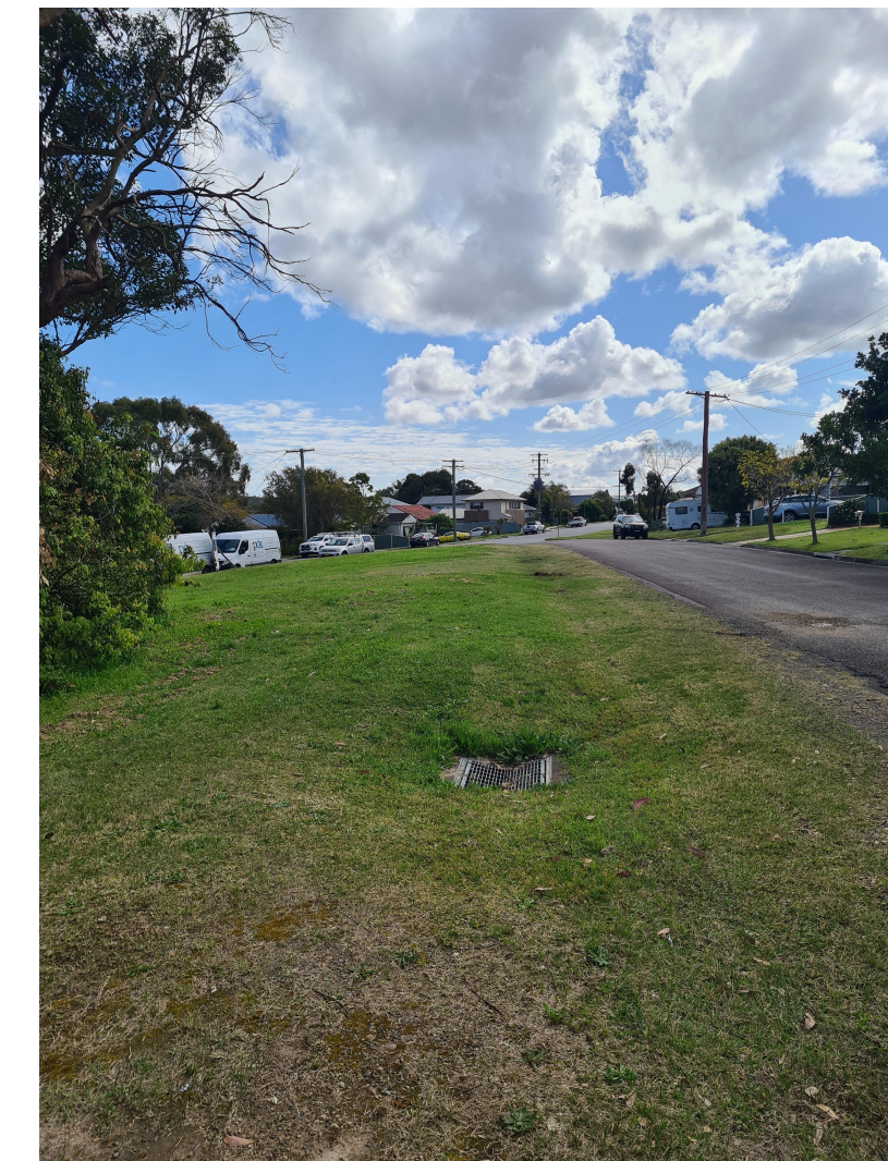
2 Existing Stormwater Drain on Holt Street
